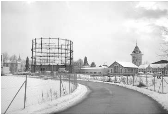
The gas works' area in Schlieren
